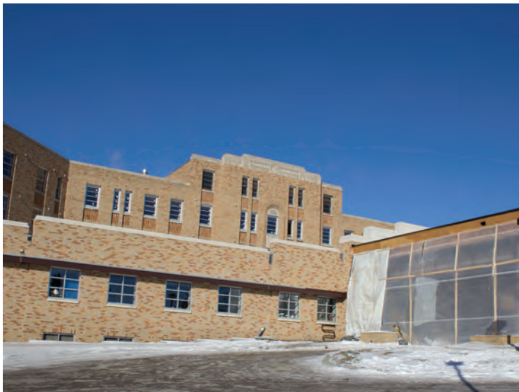
The Legacy Center under development in Jamestown, N.D.
