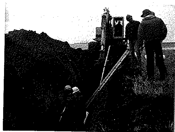
Modern trenchers and plastic pipes have made rural water systems a viable alternative to private wells.
